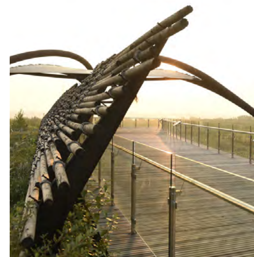
Wapisiw Lookout located at Base plant.
